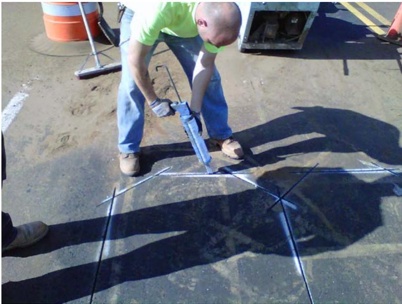
**Example F.** Sealant being installed without spillage.
