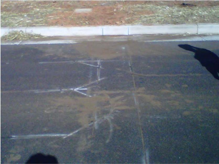
**Example G.** Each lead in has a separate cut out to the curb and are drilled through the curb.
