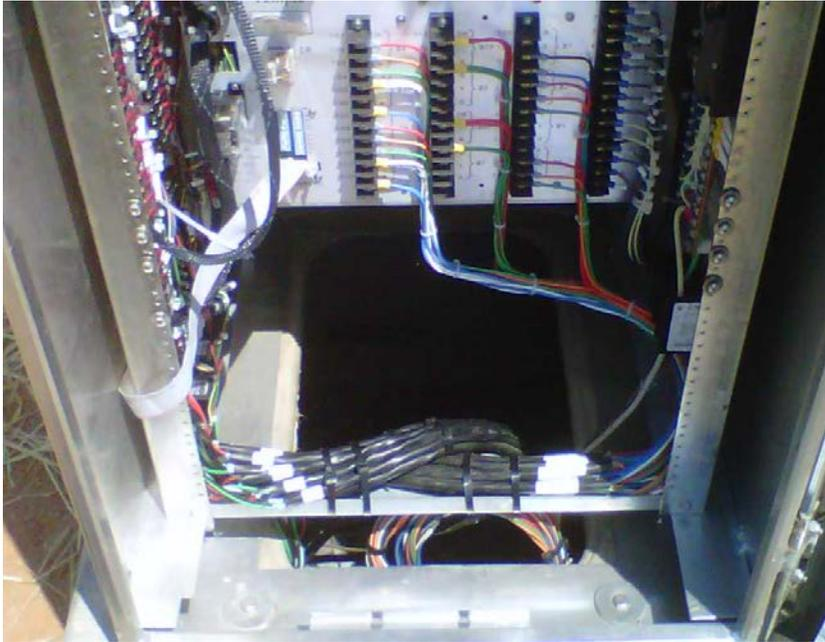
**Example C.** Notice that the wiring is cut to length and neatly terminates on each terminal. This is the only accepted method for wiring the cabinet.
