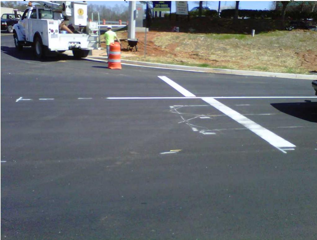
**Example H.** The nose of a loop passing the stop bar by only 24".
