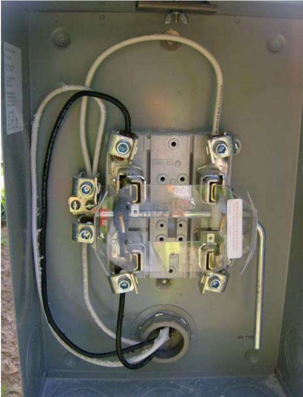
Example. B. proper wiring of a meterbase
